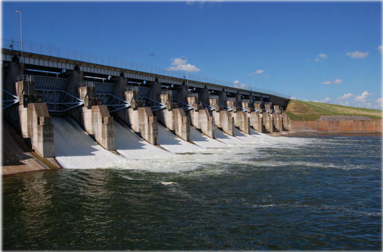
LAVON LAKE DAM
