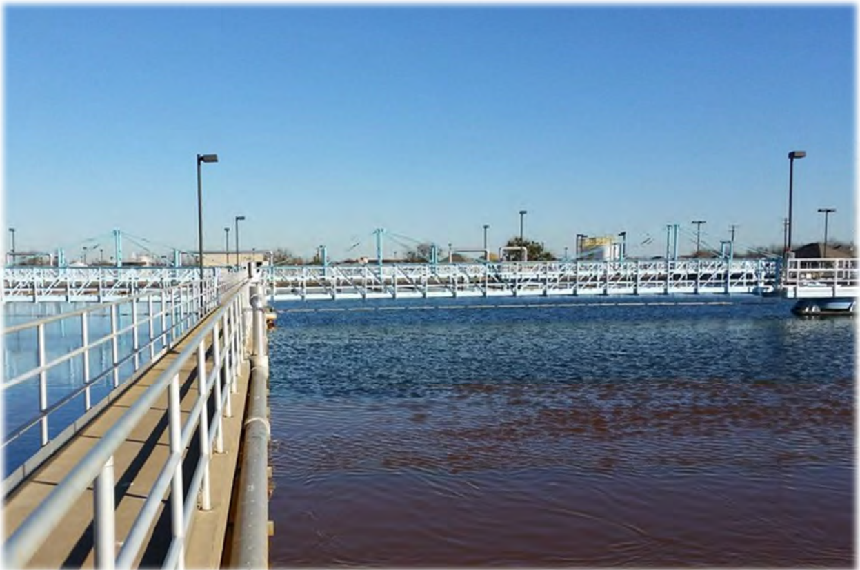
WYLIE WATER TREATMENT PLANT
