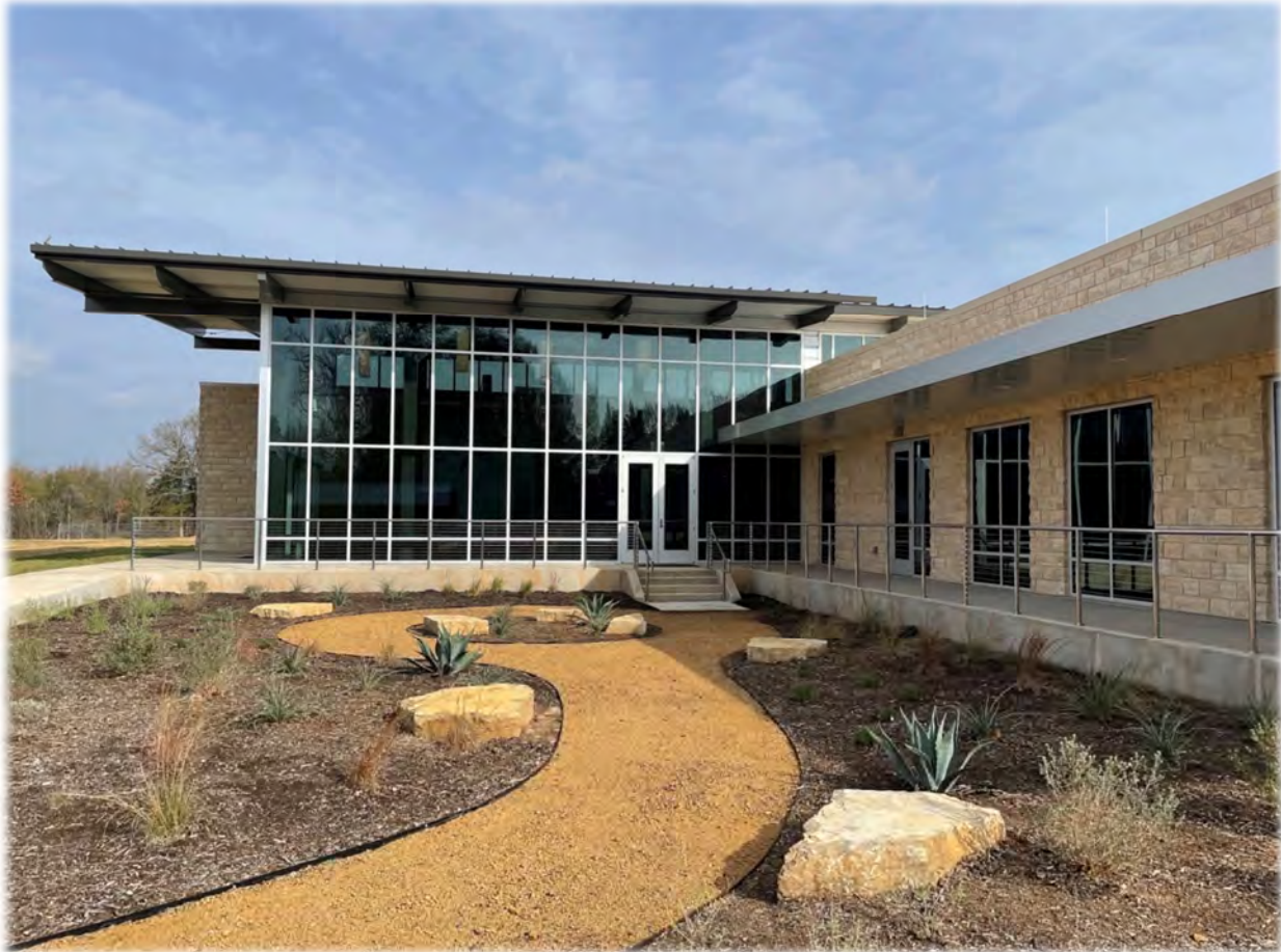
BOIS D'ARC LAKE OPERATIONS CENTER
